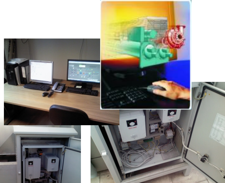
Rational space ventilation: Redesign ventilation in 2 fresh air handlers
